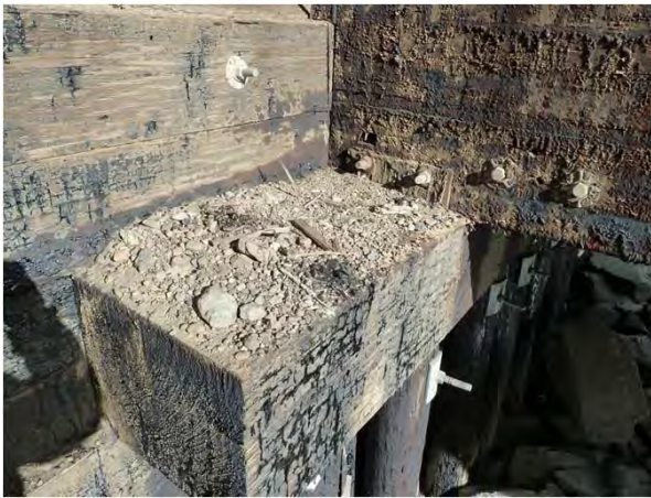
Figure 1-13: Upstream camp end cap beam.
