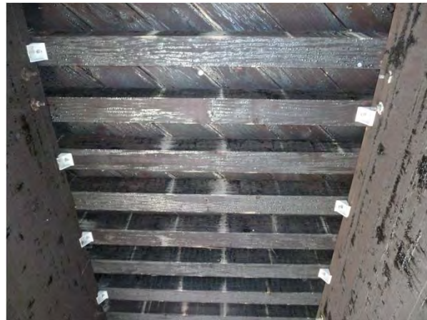
Figure 1-8: Typical underside of deck.
