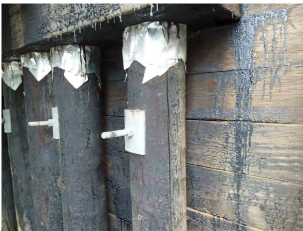
Figure 1-11: Camp end pile #8.
