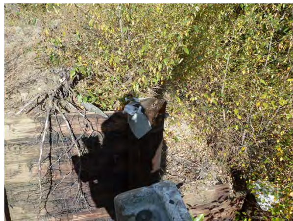
Figure 1-12: Downstream camp end soldier pile.
