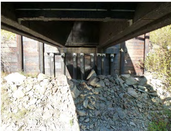
Figure 1-9: Camp end abutment.
