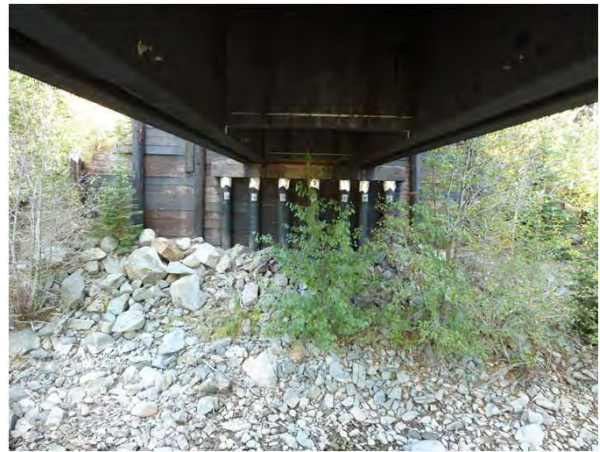
Figure 1-14: Woods end abutment.
