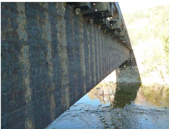
Figure 1-17: Downstream face of girder 2.
