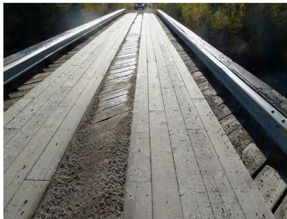
Figure 1-6: Typical deck condition.
