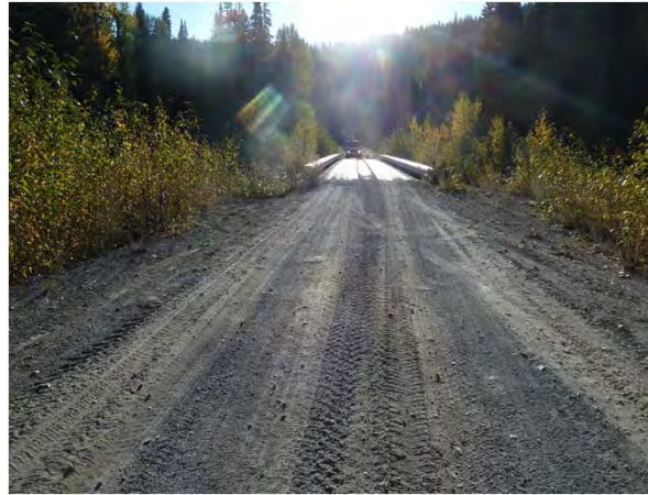
Figure 1-2: Looking towards woods end.
